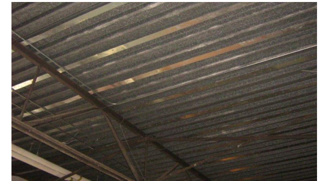
Steel deck diaphragm
