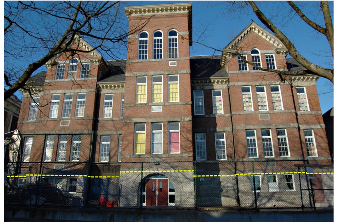
Base Isolation upgrade of 120 year old school building; plane shown by dashed line
