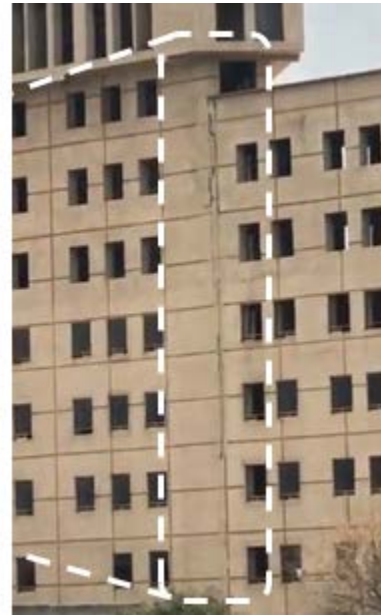
Figure 8.4. Damage produced by pounding at Hotel Miled located in the Metepec municipality, Mexico State (QuieroTV, 2020).
