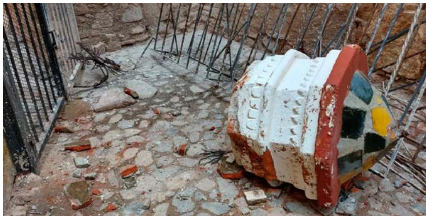
Figure 7.24. Collapse of ornamentation in the San Mateo Macuilxóchitl church in the Tlacoahuaya, Oaxaca (Guerrero en Vivo, 2020).
