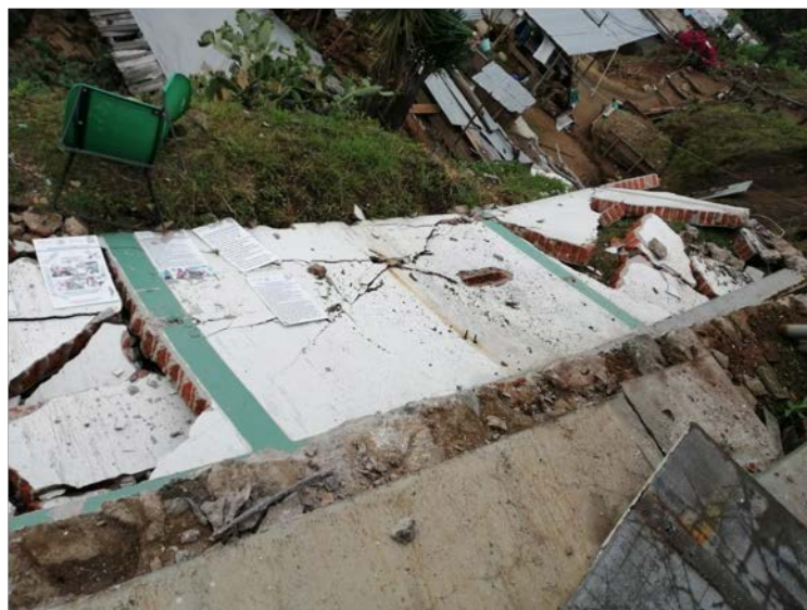
Figure 7.18. Failure of unreinforced masonry wall of the medical unit located at Santa Catarina Xanaguía in the San Juan Ozolotepec municipality, Oaxaca (Twitter, 2020I).
