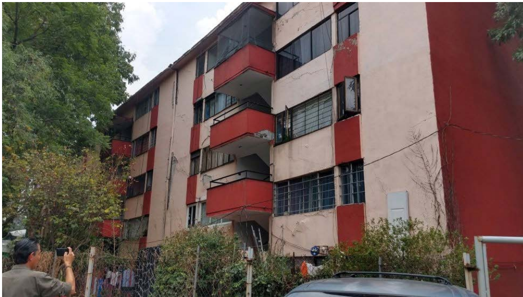
Figure 8.1. Apartment building tilted at Unidad Habitacional Lindavista-Vallejo in Mexico City (Lopez-Doriga, 2020).
