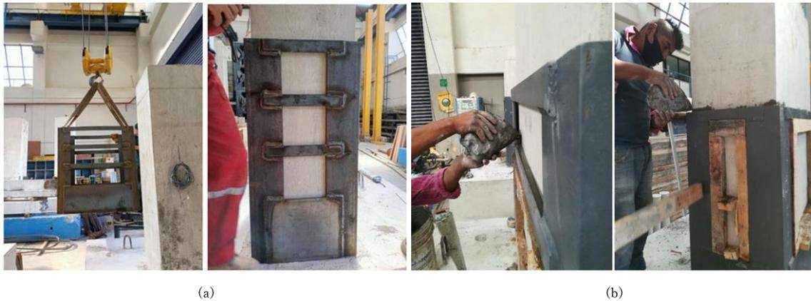
*Fig. 3.10—(a) lifting and placed of pre-armed steel jacket; (b) pouring of Sika grout*
