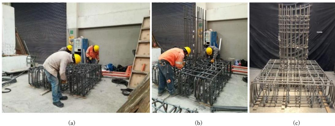
*Fig. 3.5—Steel work: (a) foundation; (b) column; (c) final work*
