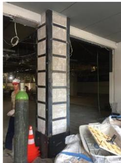
**Fig. 1.2—Steel jacketing in a column using steel angles and battens (Stelios, 2023)**
