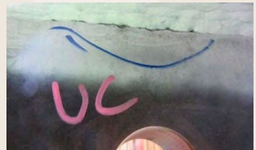
Figura 8.2.5.e Socavación del material base. Fuente: https://technoweld.com.au/2019/11/13/the-most-common-welding-defects-causes-and-remedies/
