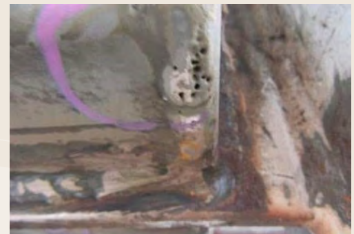
Figura 8.2.5.d Porosidad superficial en la soldadura. Fuente: https://technoweld.com.au/2019/11/13/the-most-common-welding-defects-causes-and-remedies/
