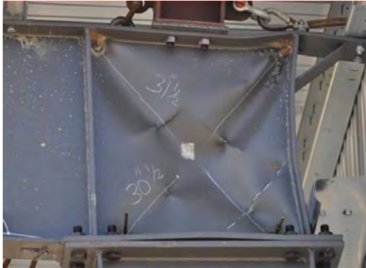
8.2.5.a.ii Rotura en zona de panel. Fuente: https://www.structuremag.org/wp-content/uploads/2014/08/0814-sp-2.jpg
